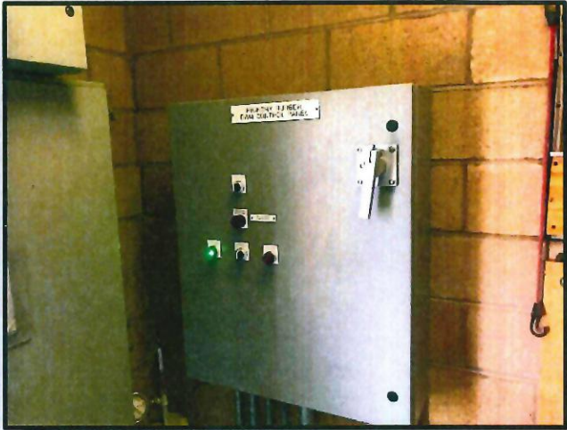
Rubber Dam control panel
